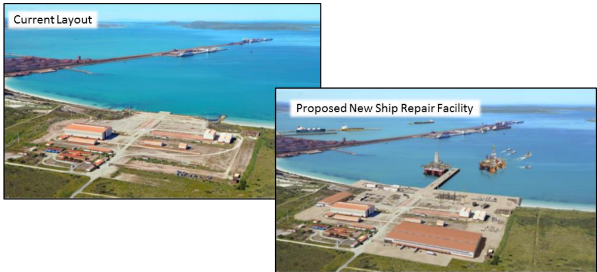
Figure 13.2.8.3 - An artist's impression of the area before and after the development of a ship repair facility in the Port of Saldanha
